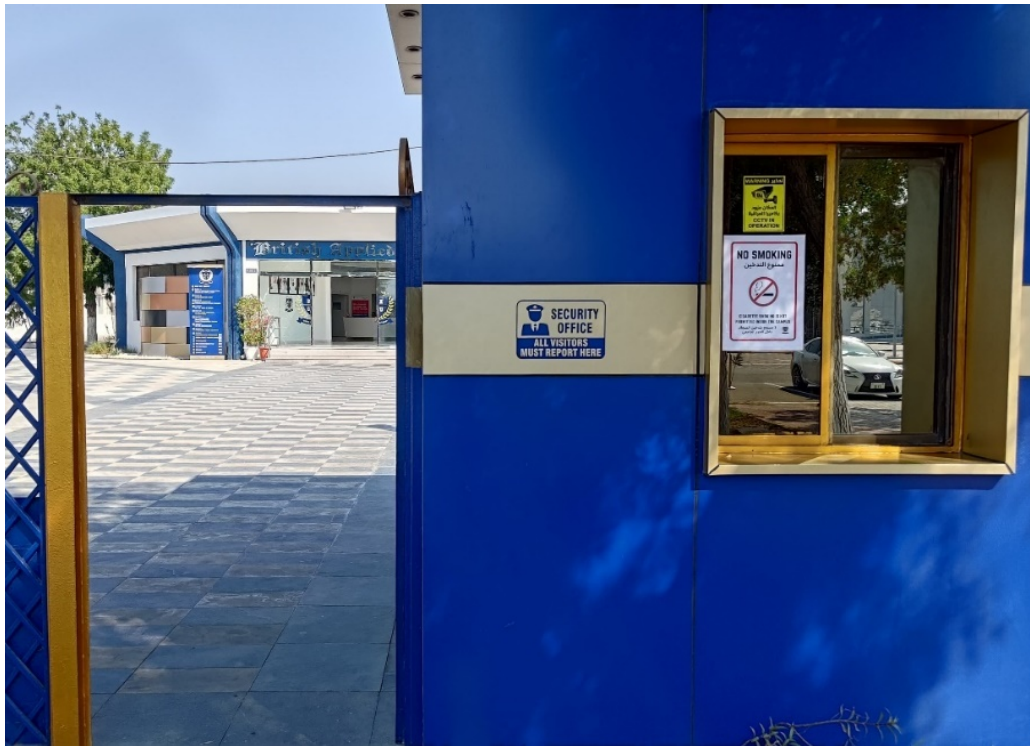
Fig 19: Security Control Room at BAC
