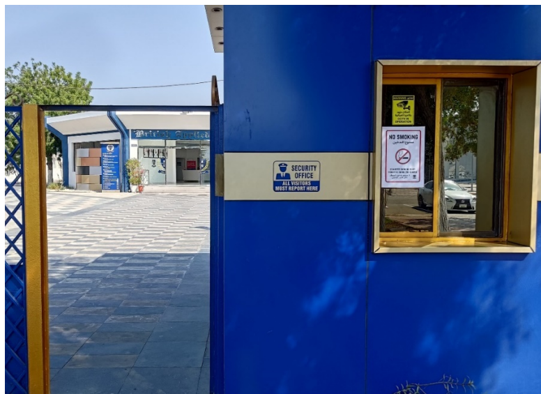
Figure 09 : Security Control Room at BACU
